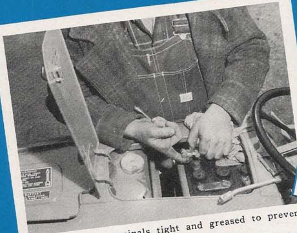
After inspecting or filling battery, always replace battery cover plate.
