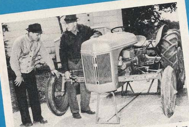
With tractor on Ferguson Power Jack, wheel spacings are easily changed.
