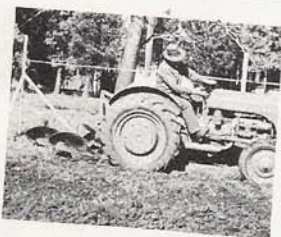
Plowing headlands. Easy turning and backing makes it possible to finish out corners neatly.
