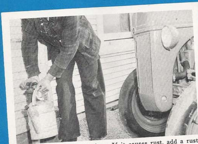
Radiator water must be clean. If it causes rust, add a rust inhibitor.
